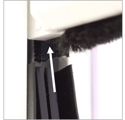
Engage the zip at the bottom of the hembar, with the opening at the centre of the plastic insert.
