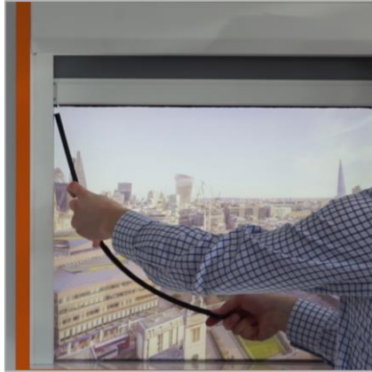
Start to slide one end of the black plastic insert up the channel with the fins facing outwards.
