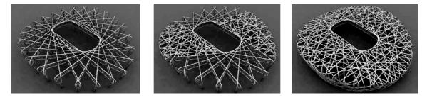
[Source: <u>http://www.structuremag.org/article.aspx?articleID=754</u>] (Left) Trussed Portal Frames Span the Stadium (Mid) Secondary Tubes Coupled with the Frames Create the Random Pattern (Right) Secondary Tubes Coupled with the Frames Create the Random Pattern
